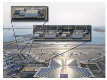
The microgrid comprises 7.66MW of rooftop solar panels, 3.68MW of fuel cells, and 2MW/4MWh of battery energy storage. Credit: Alphastruxure / PRNewswire.
